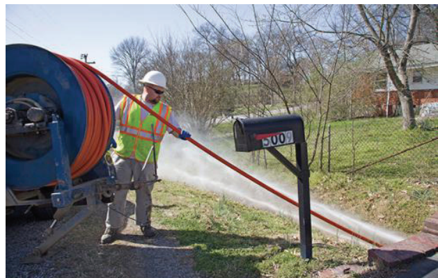
Culvert Cleaning
