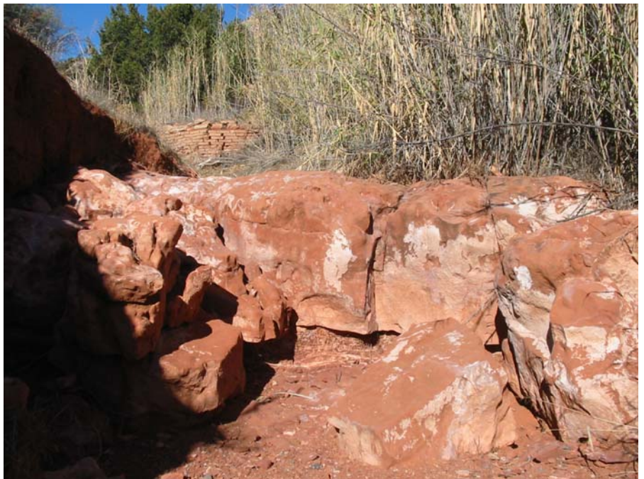
Figure 11a; Photo 2: Outcrop of weathered and broken massive to thick bedded silty-sandstone of the Supai Formation, located upstream from Seismic Survey Line HW3-S03
