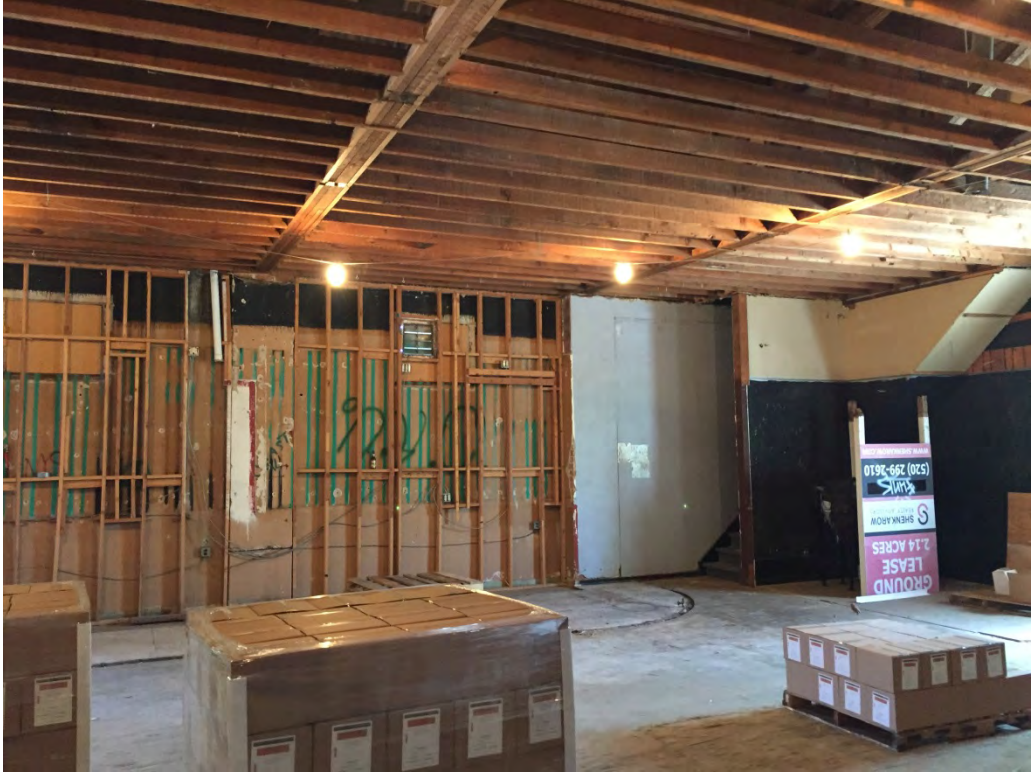
Facing Northeast toward North Building Wall
