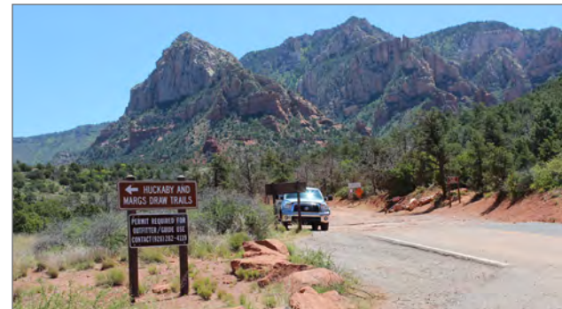
Schnebly Hill Road where the pavement ends
