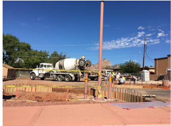
A site under development along Highway 179.
