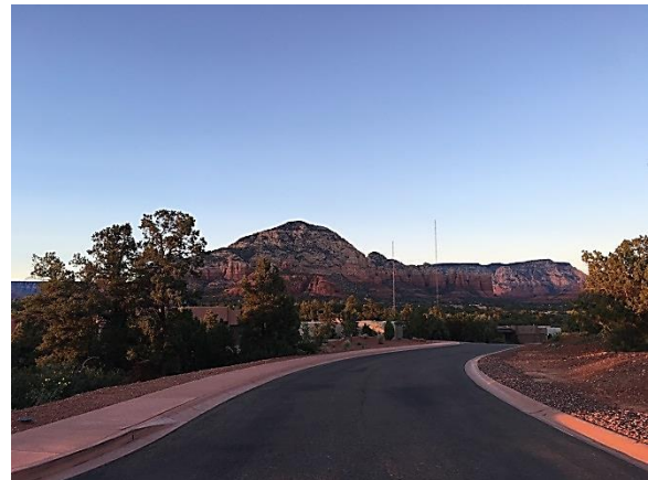
Sedona’s subdivision design standards should be clarified to address additional roadway standards and current engineering practices for new subdivisions.
