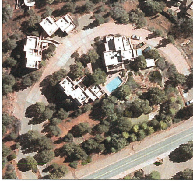
Example of a 12 unit development on less than two acres. The four buildings are clustered together leaving an open space buffer along the road.
