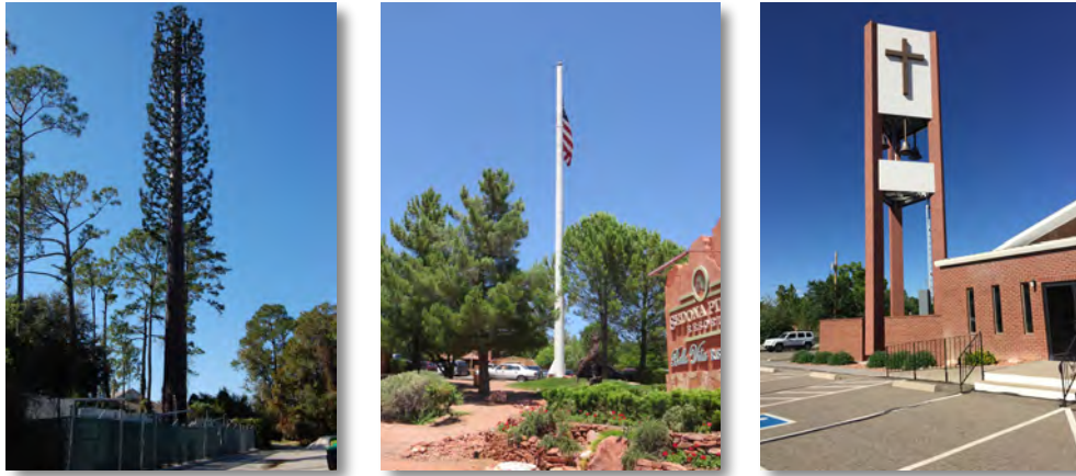
Figure 5: Concealed Macro Towers - Monopine, Flag Pole - Bell Tower
