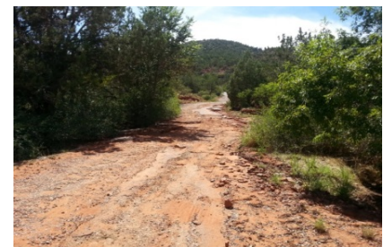
Juniper Hills Area Drainage
