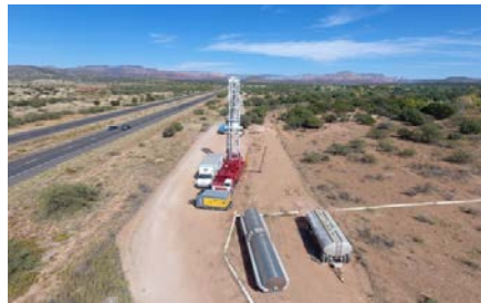
WWRP Recharge Wells
