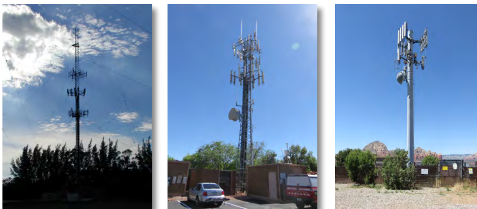
Figure 4: Non-concealed Macro Towers - Guyed - Lattice - Monopole
