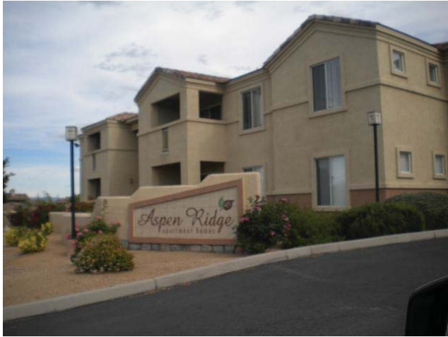
Multifamily uses in the Subject's neighborhood
