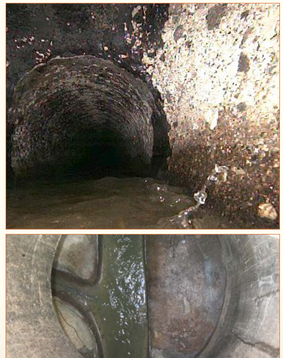
CCTV SEWER PIPE INSPECTION
