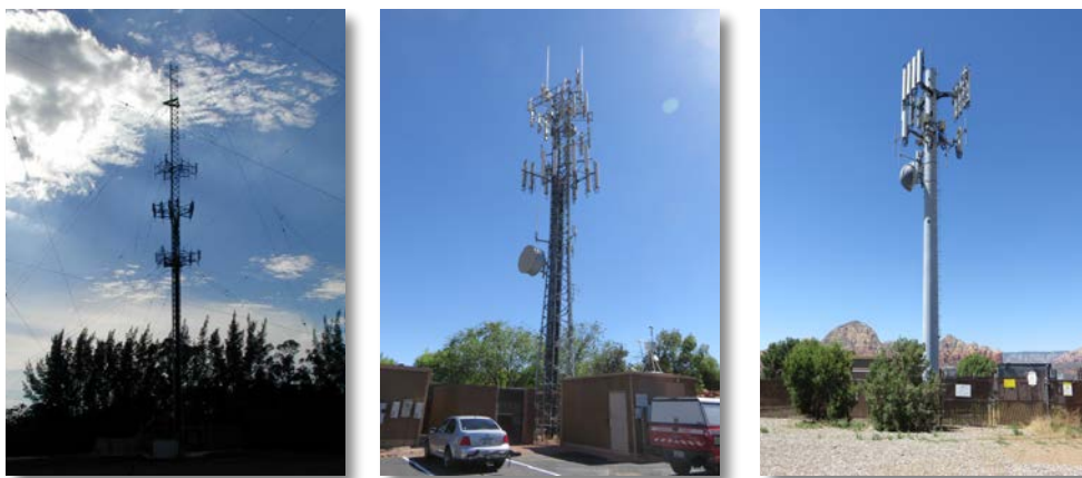
Figure 4: Non-concealed Macro Towers - Guyed - Lattice - Monopole
