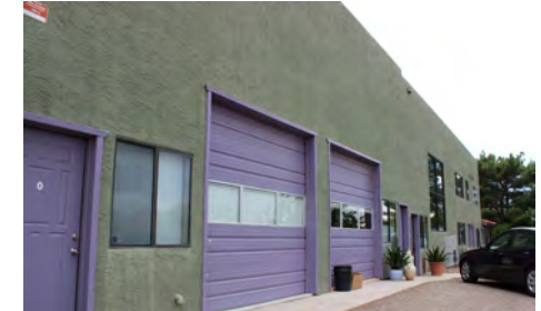
This building blends well against the hillside because of the green color and the shaded north face of the building.
