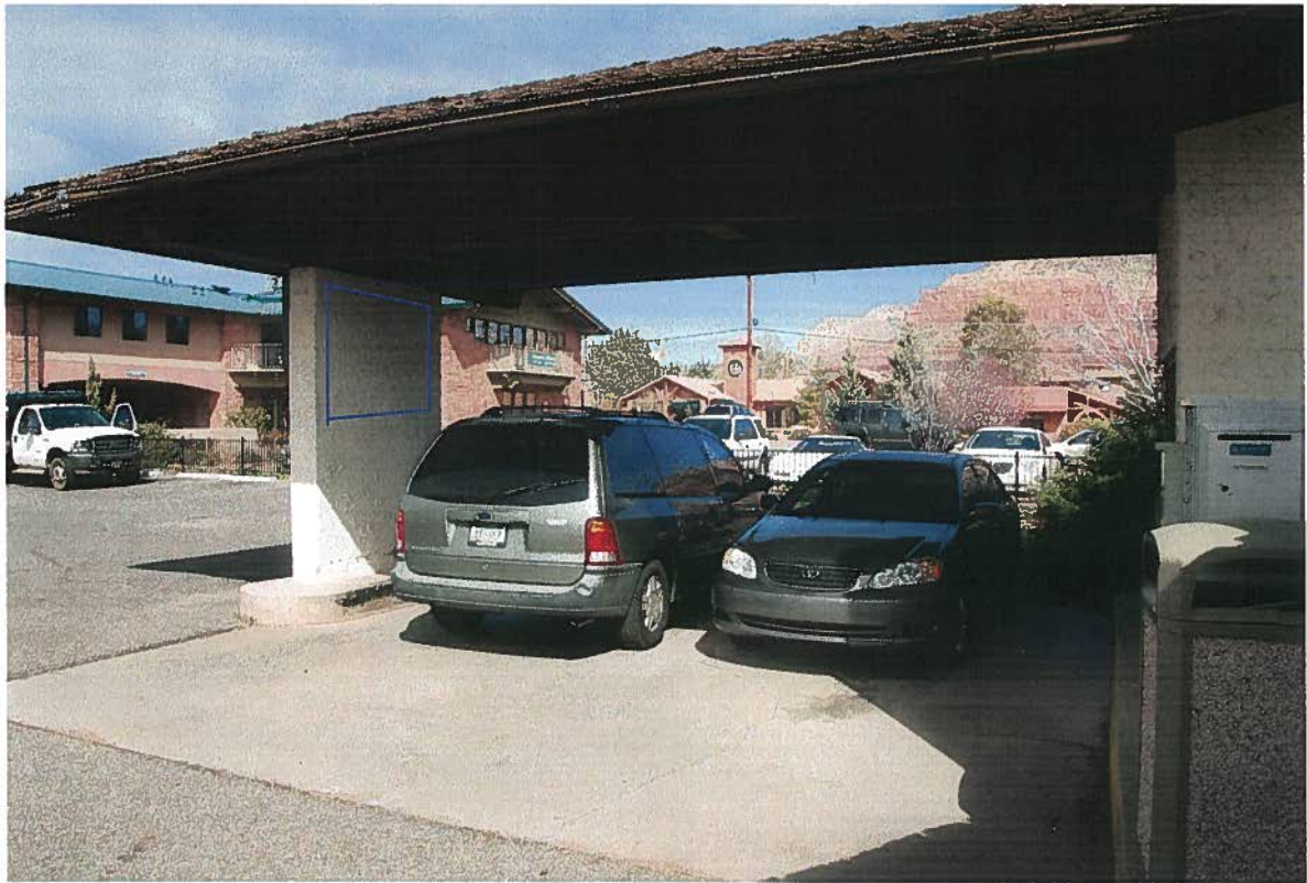
View from the rear entrance to Sacajawea Plaza. The Blue "box" on the load-bearing wall of the drive-through is the proposed site of a sign indicating "loading Zone – Red Rock Jeep"
