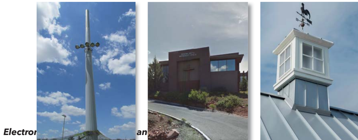
Figure 6: Concealed Base Stations - Light Stanchion - Building Concealment
