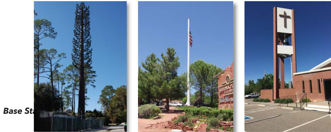
Figure 5: Concealed Macro Towers - Monopine, Flag Pole - Bell Tower
