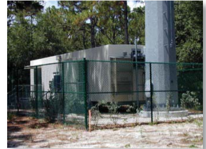
Figure 8: Low Band Facility
