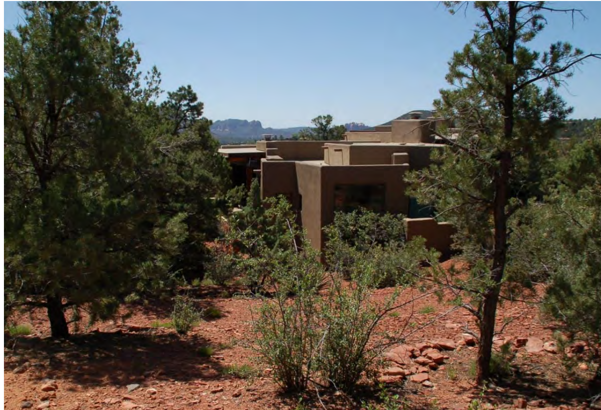
Jordan Park home adjacent to one million gallon storage tank.
