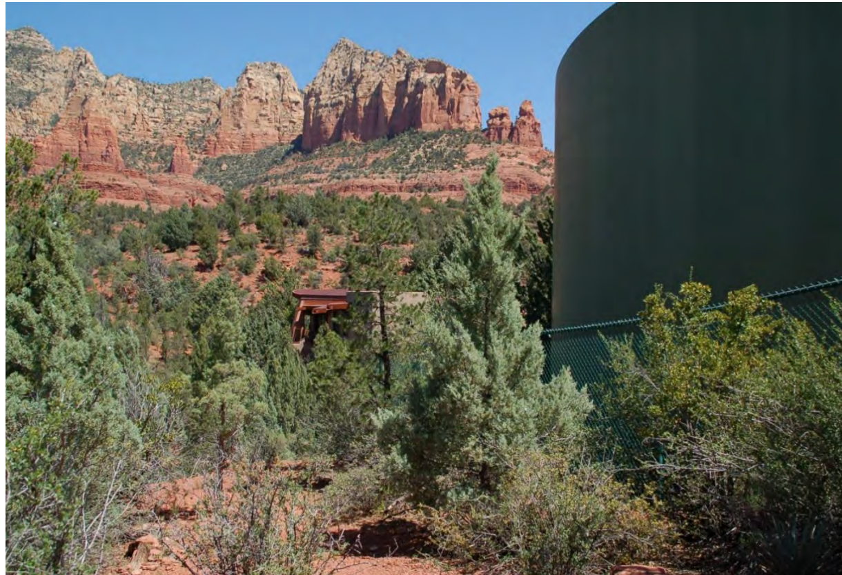
Jordan Park neighborhood, one million gallon storage tank.
