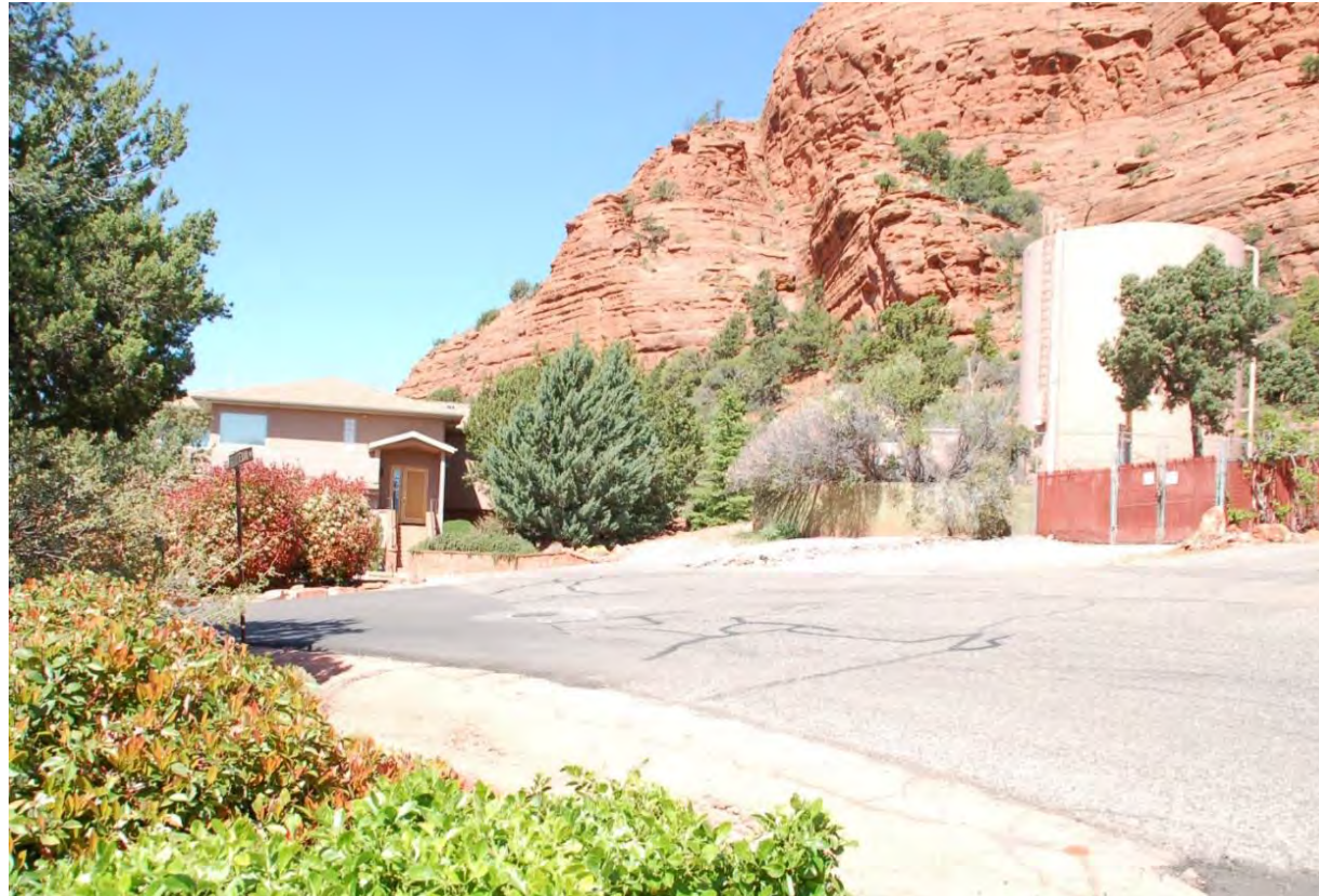
Sedona West Storage Facility, a 102,800 gallon tank between two homes.
