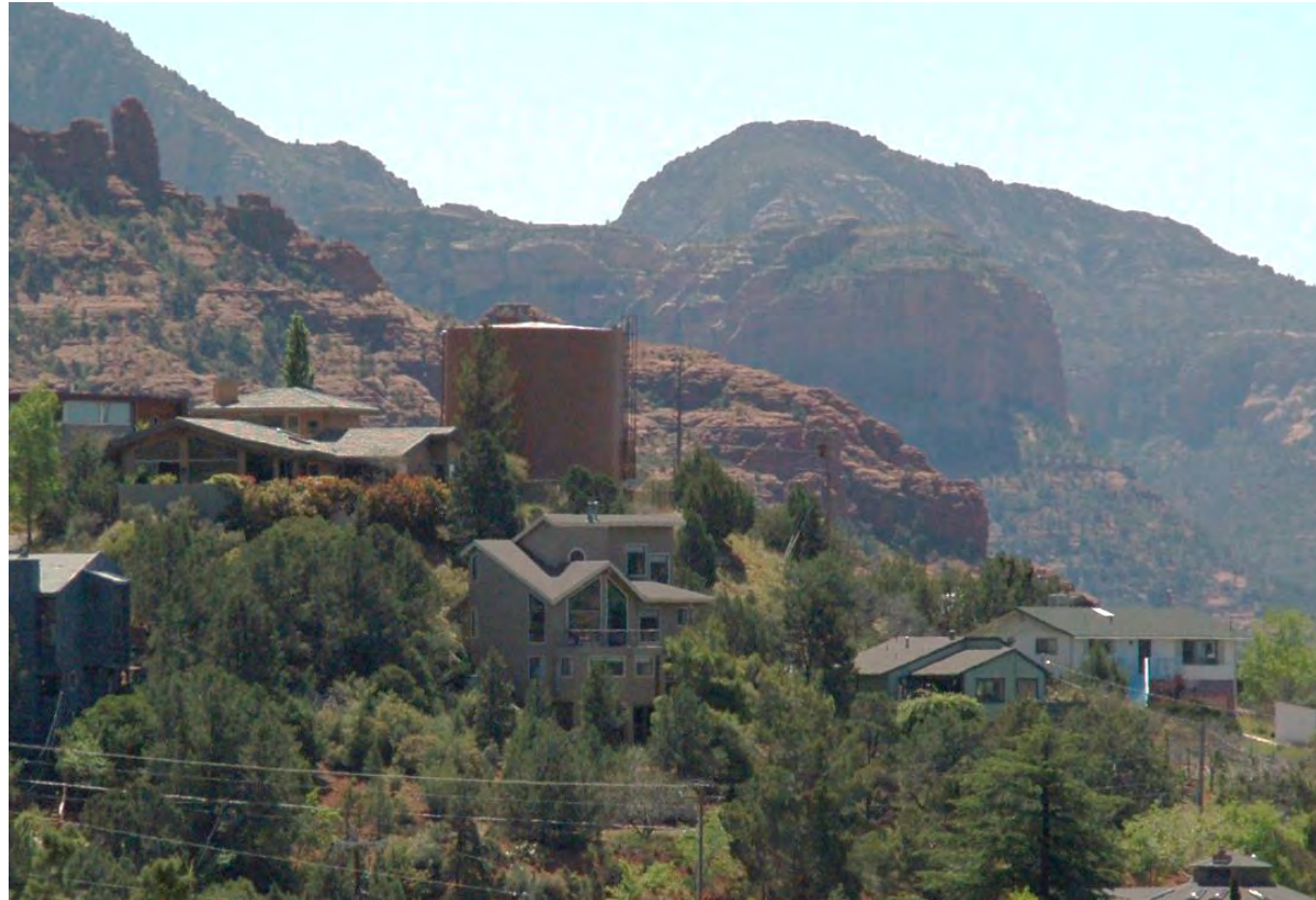
Town tank, 300,000 gallon storage tank, surrounded by homes. Homes built after tank.
