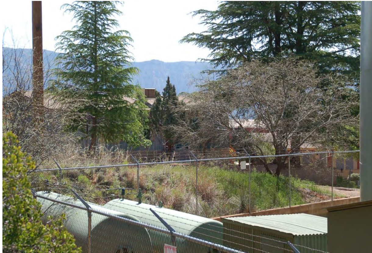
Harmony High Park, one million gallon storage tank and booster station.
