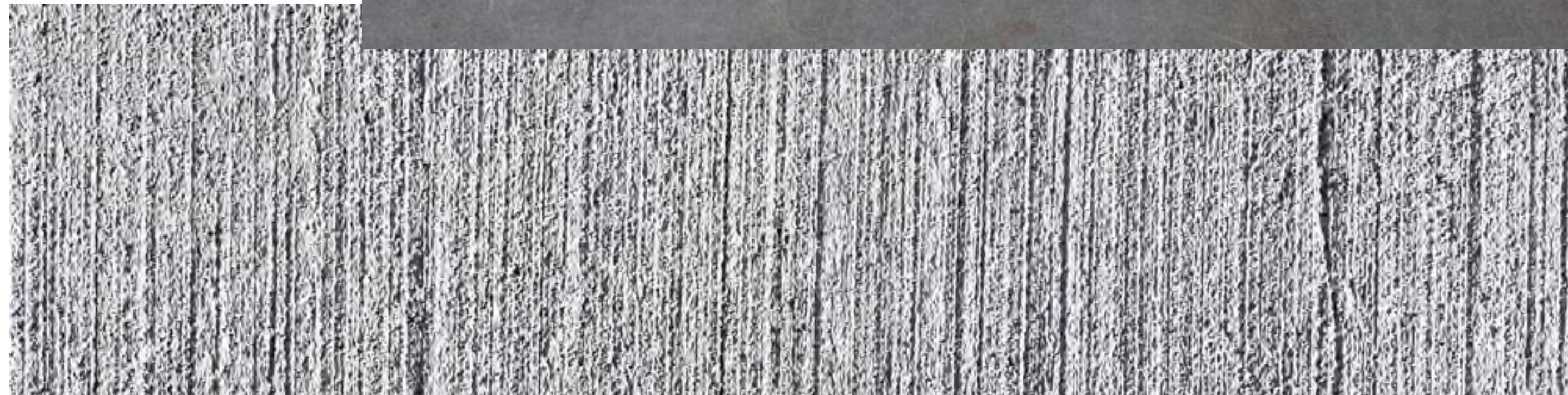
ext. concrete, broom finish
