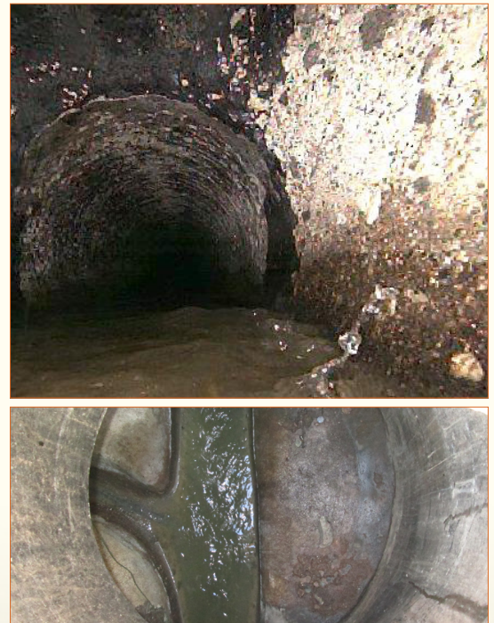
CCTV SEWER PIPE INSPECTION
