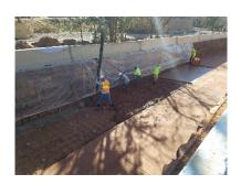
Phases 1 and 2 of this project included installing barriers along the top of the wash bank. These improvements increased the entire channel capacity between Brewer Road and Oak Creek. However, the ultimate design capacity of the channel will not be reached until Phase 4 is complete; see below.
