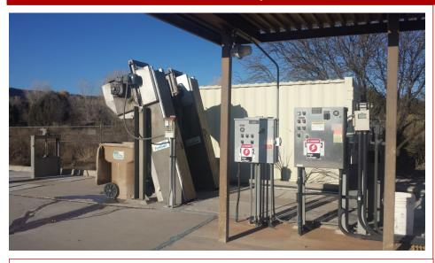
The WWRP Bar Screen & Headworks Replacement Project will replace two existing bar screens with new bar screens. The bar screens are a vital part of wastewater treatment which remove solids at the start of the treatment process.
