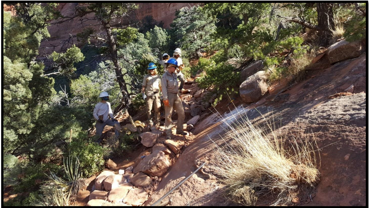
ACE working on the Hangover trail by rebuilding a switchback.
