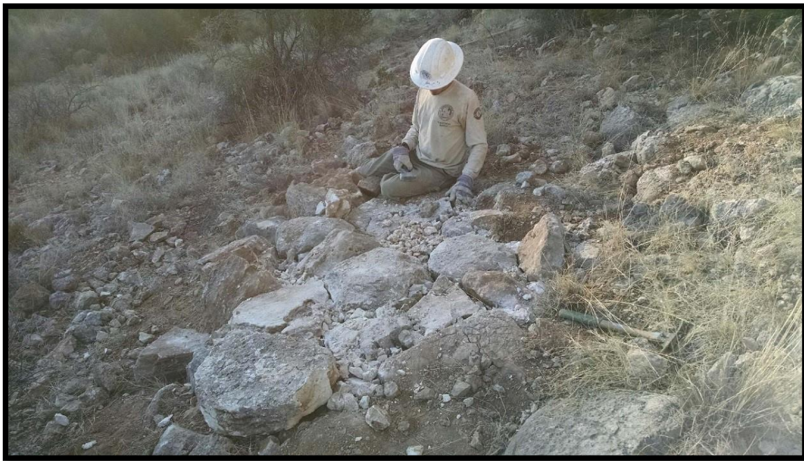
Elmore wash rock armoring project.
