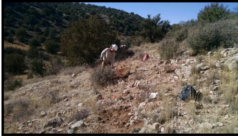
New trail construction on the Elmore Wash trail.
