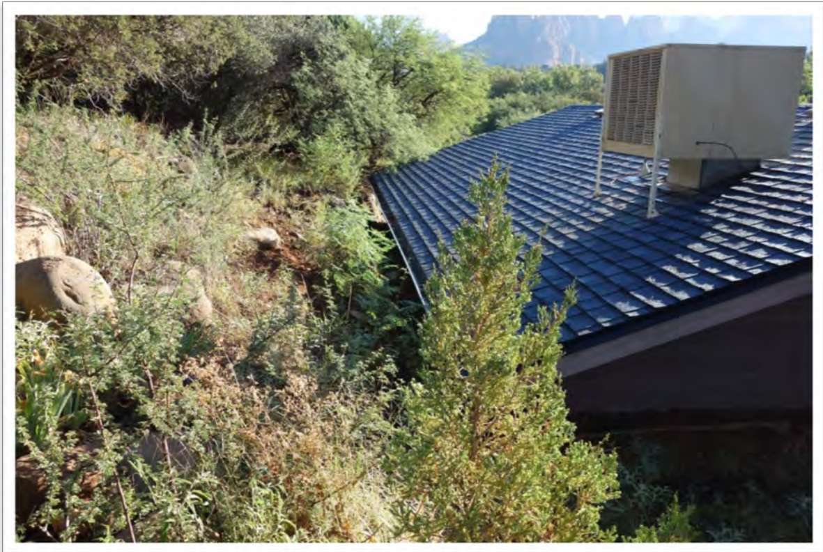
Figure 8: View of the garage from the rear property line, highlighting the
