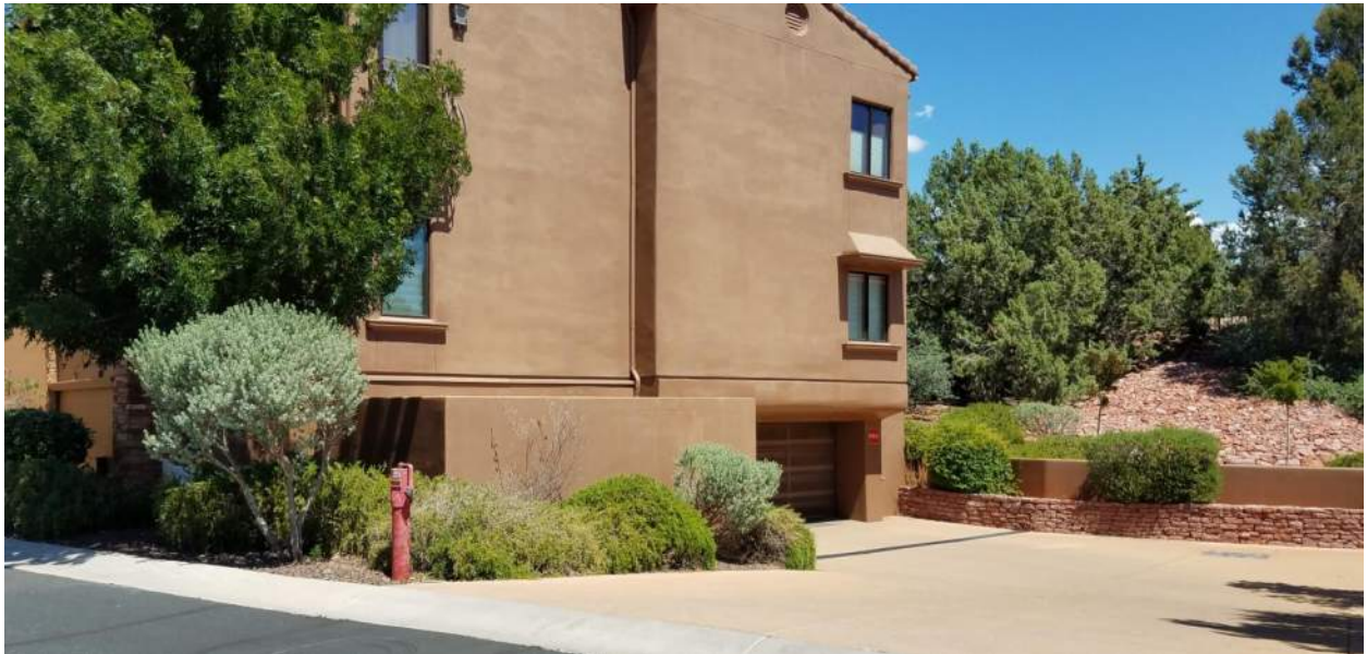
Building 109 of the existing Park Place Condominiums
