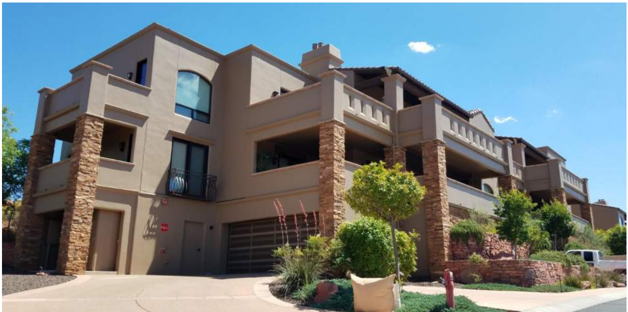
Building 110 of the existing Park Place Condominiums
