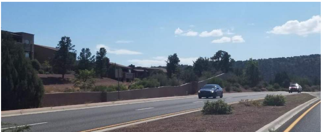
Existing conditions of the property wall & 89A frontage
