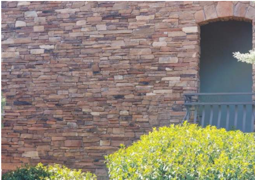
Figure 7: Building 110 Stone Veneer Elevation
