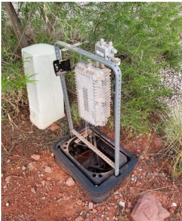
Existing cable communications utility boxes located throughout the site
