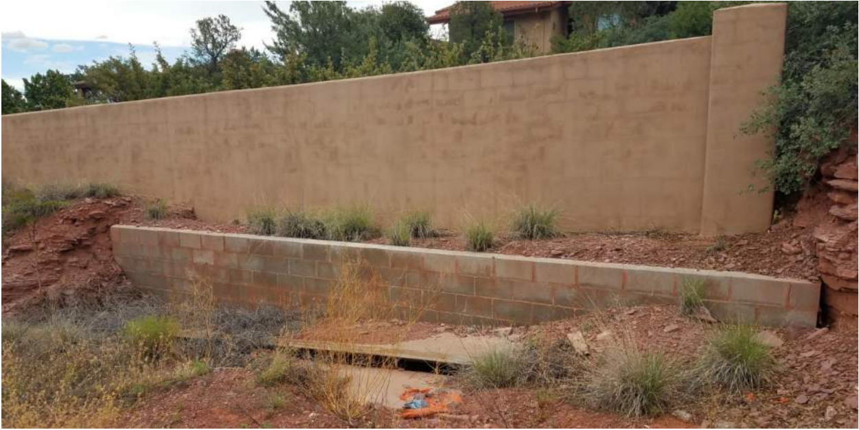
Uncompleted drainage structure on the northeast portion of the project.
