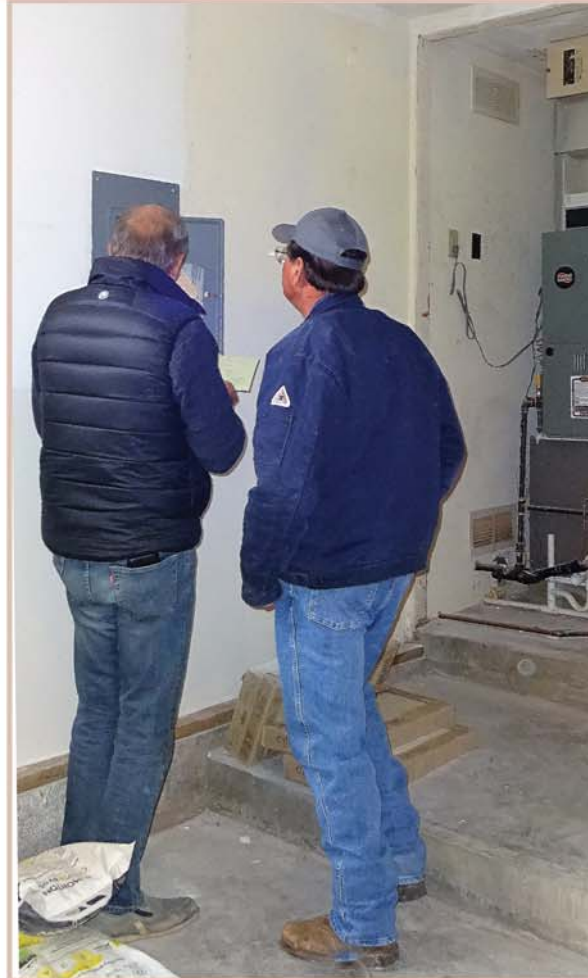
BUILDING INSPECTOR BRUCE ZOLMAN INSPECTING A RESIDENTIAL REMODEL
