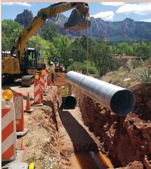
JUNIPER HILLS AREA DRAINAGE IMPROVEMENT PROJECT
