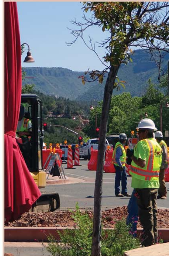
JORDAN ROAD DEMOLITION
