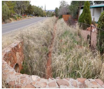
Thunder Mountain Road Existing Open Channel
