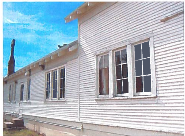
Exterior Wall - Barn
