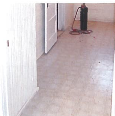
Bathroom floor - Ranger Residence
