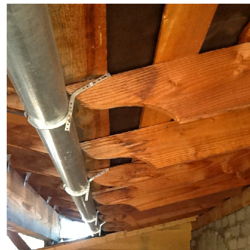
PROPOSED NEW GUTTER INSTALLATION
