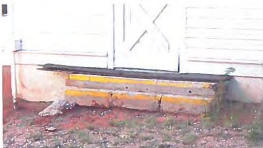
Concrete stair at the Barn
