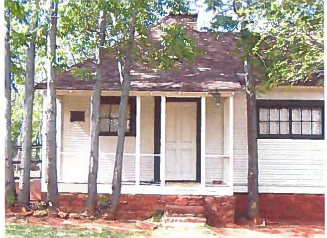
Porch railing and stair at the Ranger Residence
