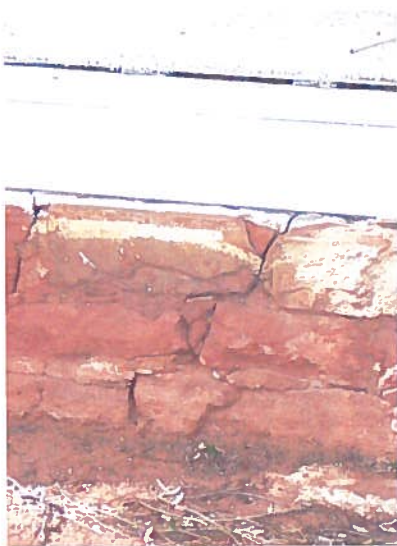
Ranger Station Residence - Sandstone Foundation
