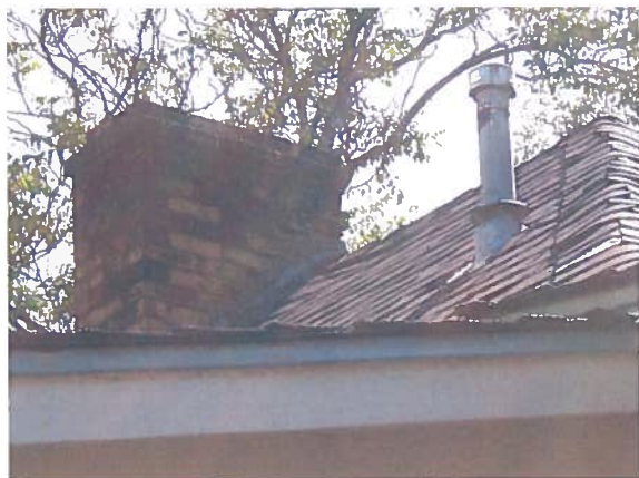
Chimney at Ranger Residence
