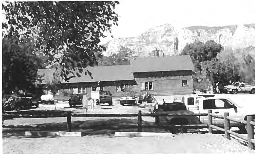
Sedona Ranger Station Barn, South Elevation - 2003 Photo Courtesy of Sedona Historical Society
