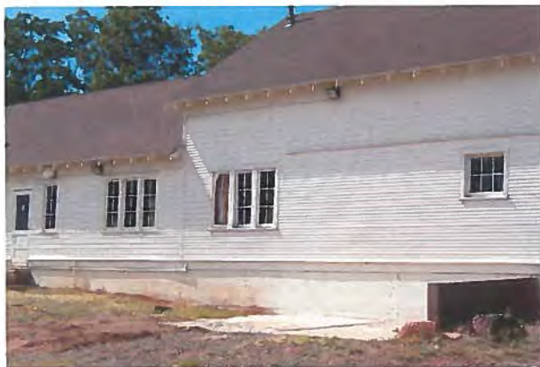
Foundation at the Barn
