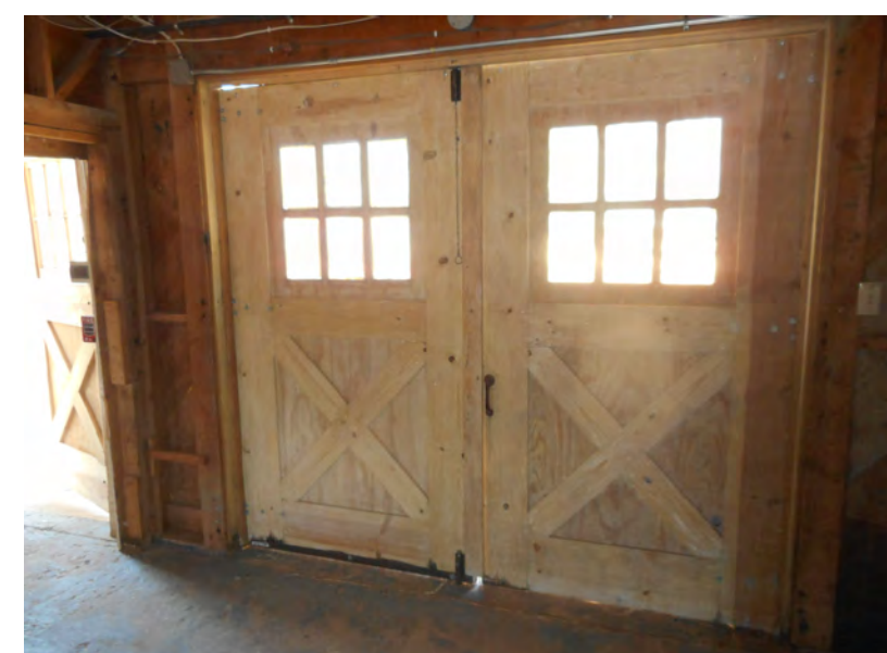
BARN EXISTING INTERIOR CONDITIONS
