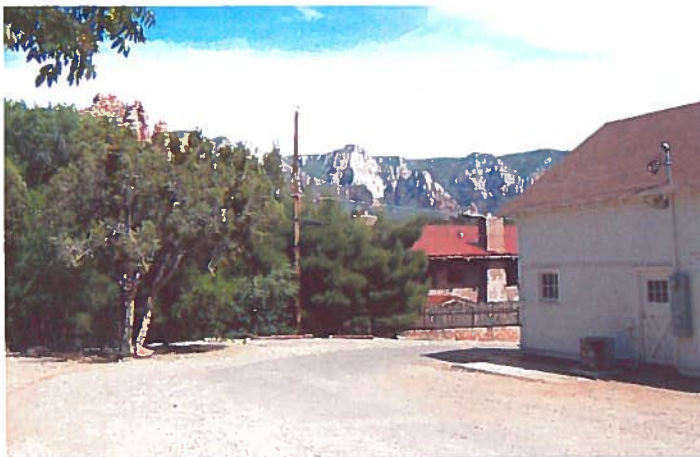
Sedona Ranger Station site, looking southeast
