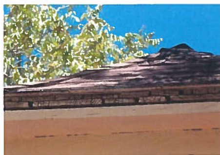
Composition roof over wood shingles at the Ranger Residence
