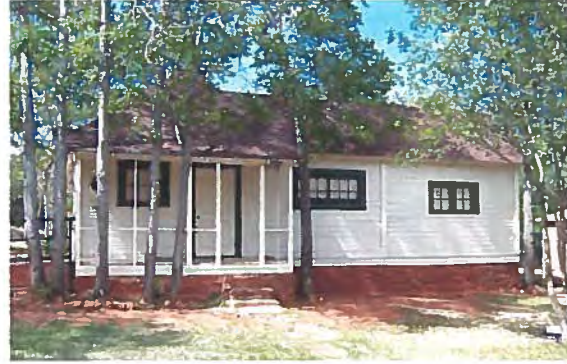
South Elevation of the Ranger Residence
