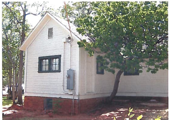
Northeast corner of the Ranger Residence
