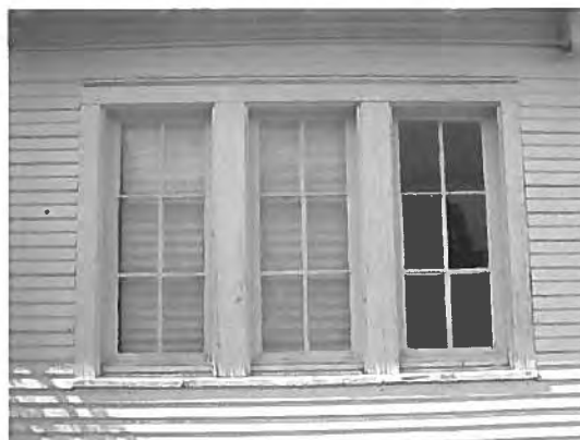
Triple casement window - Barn
