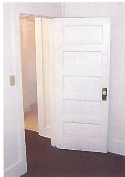
Five panel door in the Ranger Residence
