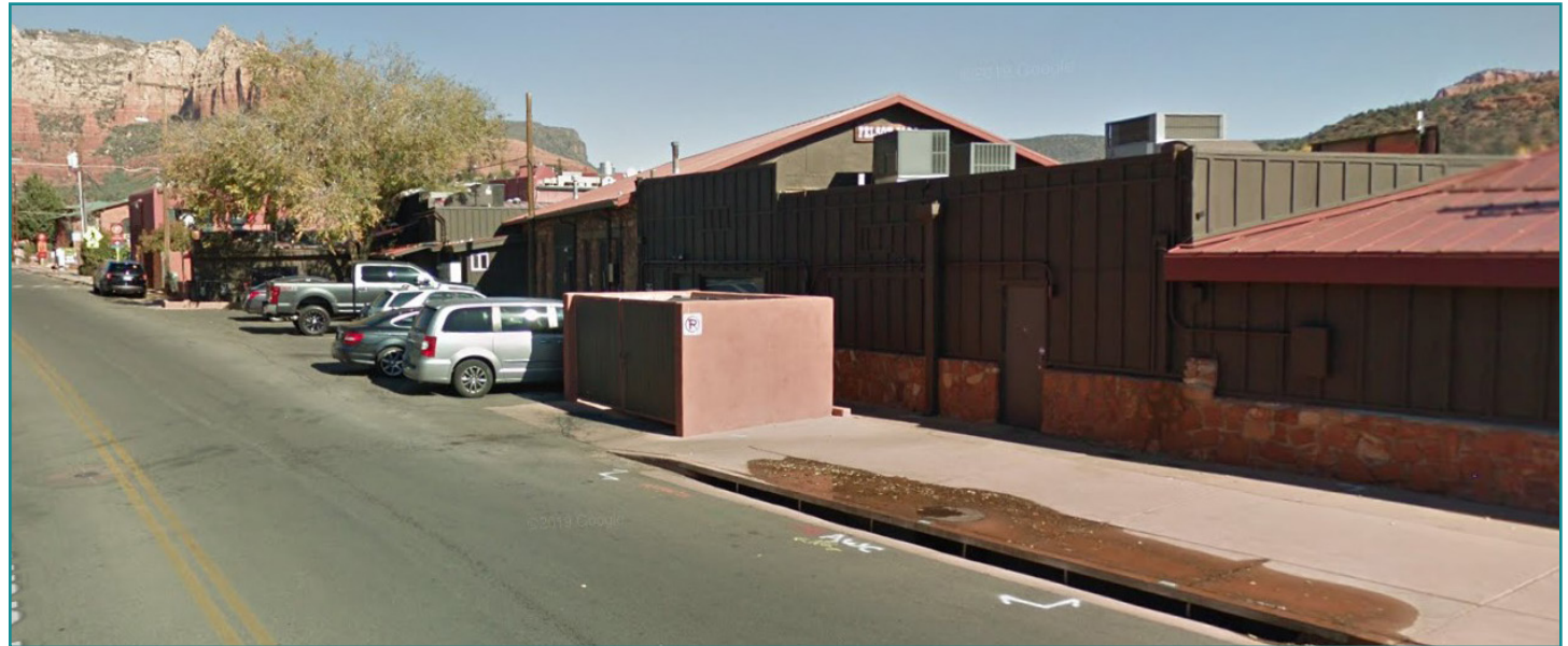
Fig 3.3. Photograph of Jordan Rd north of the roundabout.
