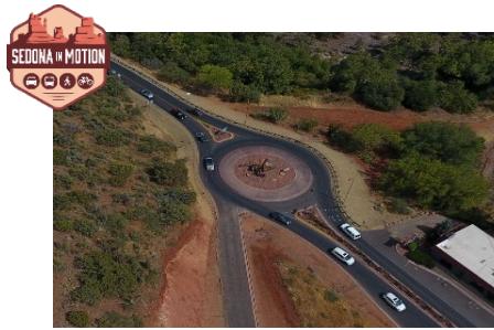
SIM 1 -Uptown Roadway Improvements
