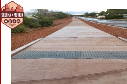
SIM 11G - Thunder Mountain/ Sanborn SUP and Drainage Improvements
