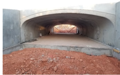
Sunset Drive Crossing Drainage Improvements
