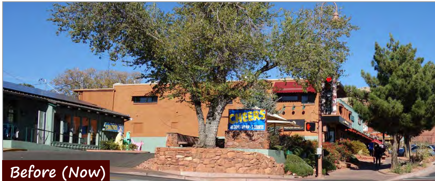
Figure 1.2. Photograph of the northwest corner in 2020.
