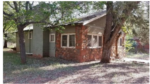
East side of Residence
