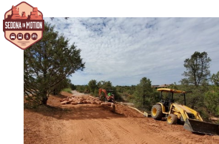
SIM 11I - Dry Creek Road Shared Use Path
