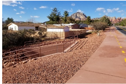
Sunset Drive Crossing Drainage Improvements
