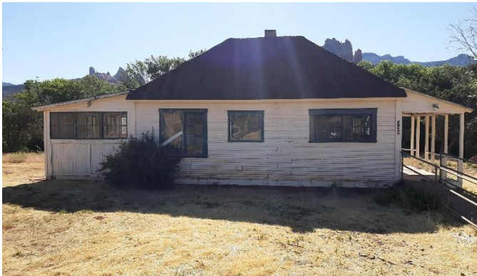
Ranger Station House (Before Restoration)
