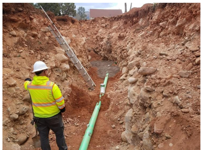
Sewer Utility Work
