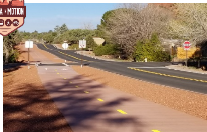
SIM 11G - Thunder Mountain/ Sanborn SUP and Drainage Improvements
