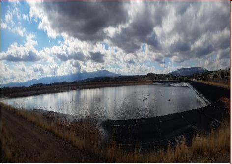
The Wastewater Department storage treated wastewater in a 70 million gallon reservoir prior to sending the water to irrigation as part its effluent management strategy. The reservoir is lined to prevent seepage in a 70 million gallon earthen reservoir. The existing liner is original to the construction of the reservoir and is necessary to maintain compliance with the Arizona Department of Environmental
