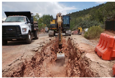
Shelby Drive Roadway Improvements
