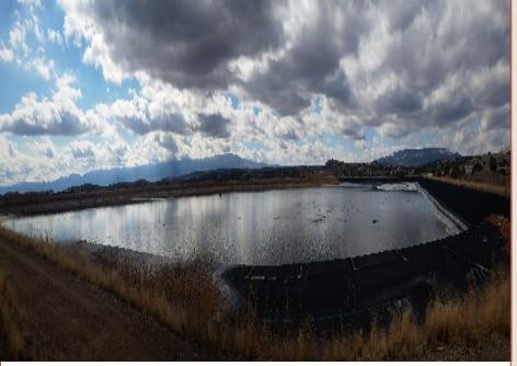
The Wastewater Department storage treated wastewater in a 70 million gallon reservoir prior to sending the water to irrigation as part its effluent management strategy. The reservoir is lined to prevent seepage in a 70 million gallon earthen reservoir. The existing liner is original to the construction of the reservoir and is necessary to maintain compliance with the Arizona Department of Environmental Quality. This project will replace the liner.
