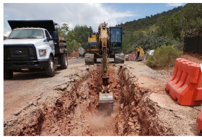
Shelby Drive Roadway Improvements
