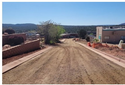
Shelby Drive Roadway Improvements
