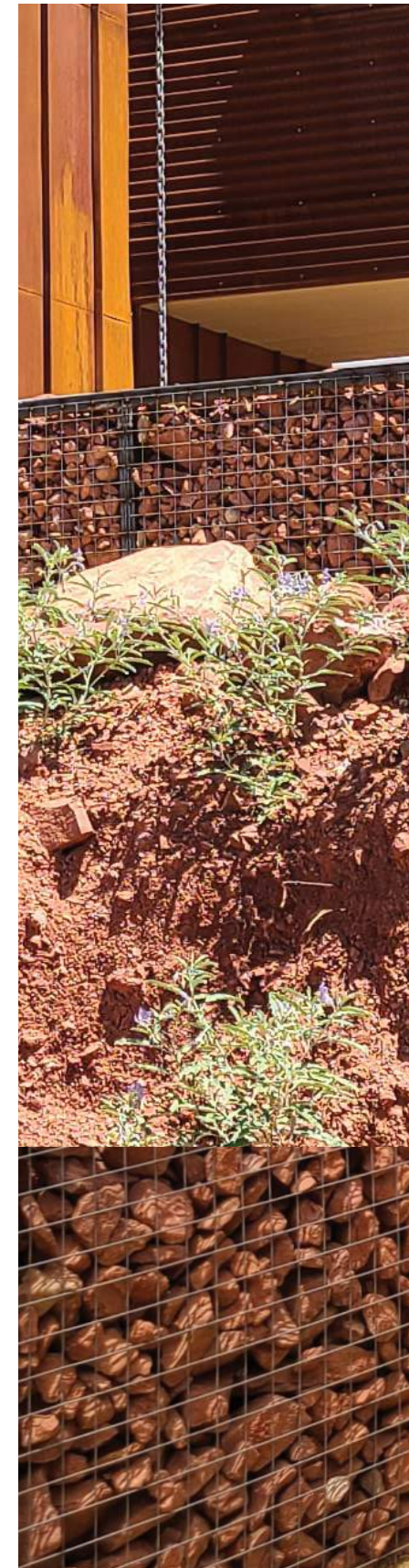
SITE WALLS SITE HARVESTED BOULDERS OR GABIONS
