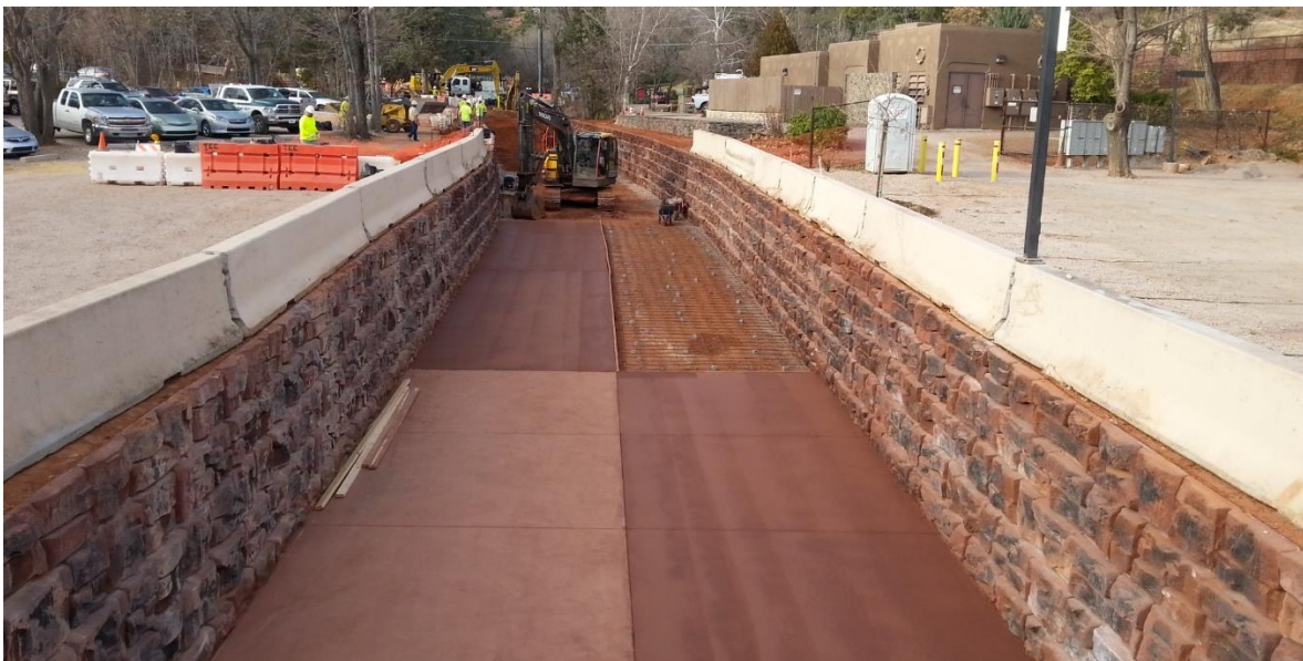
Figure 3-6 Soldier Wash Channel Construction
