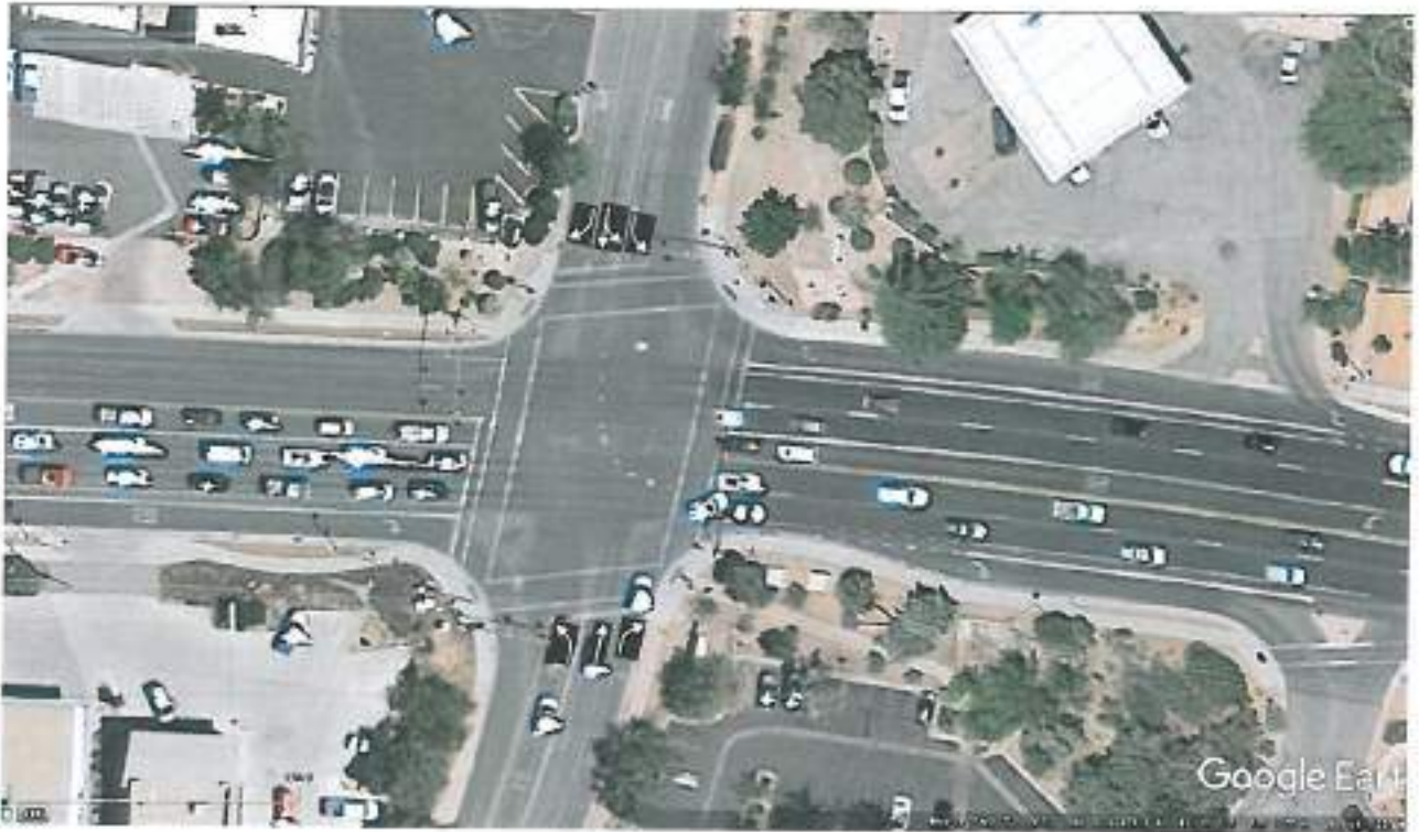
Existing N/S Lane Configuration and Intersection Pavement Markings
