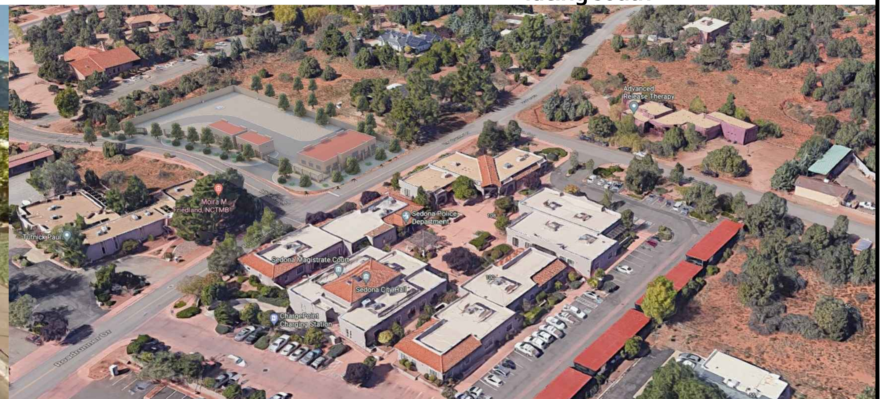
① facility birds eye view southeast corner
