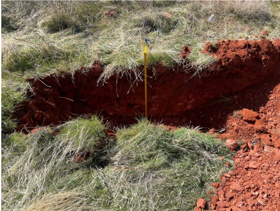
Photo 19 – Excavated Test Pit 10. Test Pit 10 was terminated at a depth of 2.0 feet due to backhoe refusal on hard mudstone bedrock. The red soils encountered to a depth of 1.0 feet consist of red silty sandy gravel with cobbles, medium dense, damp, low PI. From 1.0 to 2.0 feet, the soils became lighter in color, clayey silty gravel with cobbles, some sand, dense, slightly damp, PI of 5, probable highly weathered mudstone bedrock.
