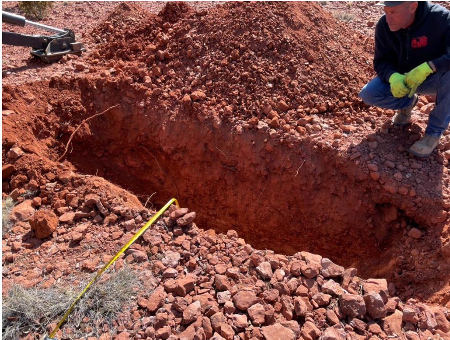
Photo 1 – Excavated Test Pit 1. Test Pit 1 was terminated at a depth of 4.0 feet due to backhoe refusal on hard mudstone bedrock. The soils encountered to a depth of 1.5 feet consist of red sandy gravelly silt, stiff, slightly damp, low PI. From 1.5 to 4.0 feet, the soils became lighter in color and dense, probable highly weathered mudstone bedrock.
