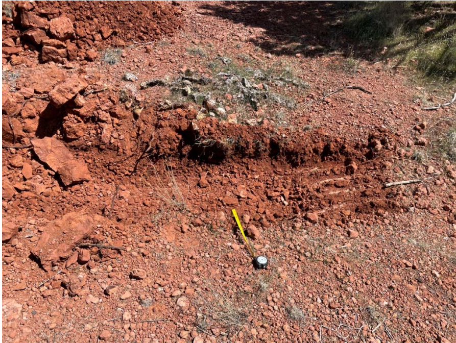
Photo 9 – Excavated Test Pit 5. Test Pit 5 was terminated at a depth of 1.0 feet due to backhoe refusal on hard mudstone bedrock – Supai Formation. . The upper 1.0 feet of red silty gravel with sand and cobbles is medium dense, damp, PI of 2 .
