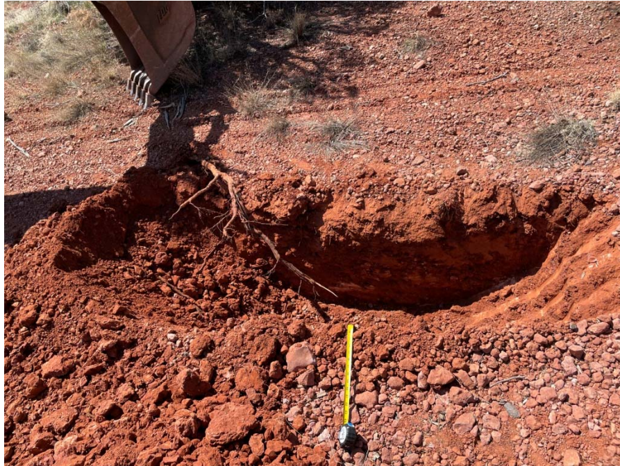
Photo 7 – Excavated Test Pit 4. Test Pit 4 was terminated at a depth of 2.0 feet due to backhoe refusal on hard mudstone bedrock – Supai Formation. . The upper 2.0 feet of red clayey silty gravel with sand and cobbles are medium dense, damp, PI of 5.
