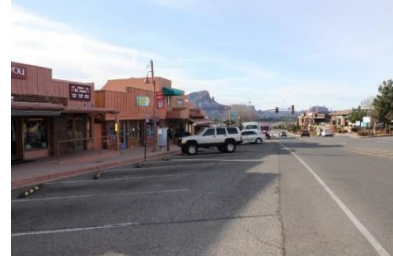
SR 89A in Uptown Sedona includes on-street parking, one lane in each direction, and a continuous two-way left turn lane. North of Uptown, SR 89A transitions to a two-lane rural roadway as it enters Oak Creek Canyon.
