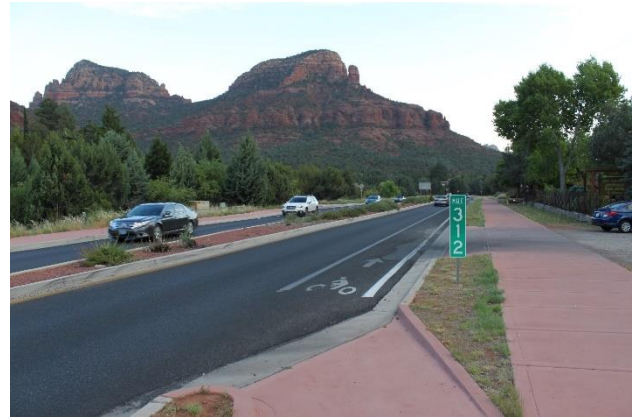
SR 179 at MP 312. SR 179 consists of one lane in each direction, a raised median, and a bicycle lane.
