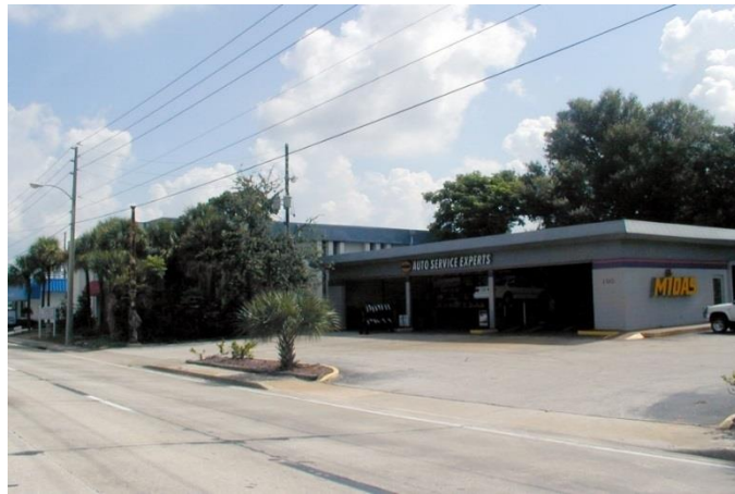
Property with two closely spaced driveway openings
