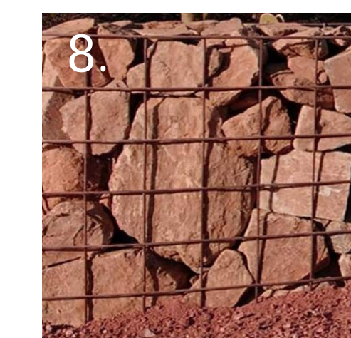
8. Red Rock Gabion Walls
