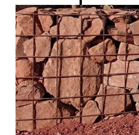
Red Rock Gabion Walls
