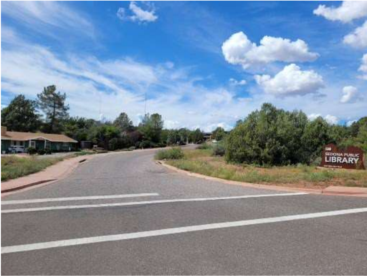
White Bear Road/ Dry Creek Road Intersection (the path will be on the right side, or north side of White Bear Road)
