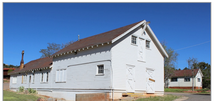
Ranger Station Barn
