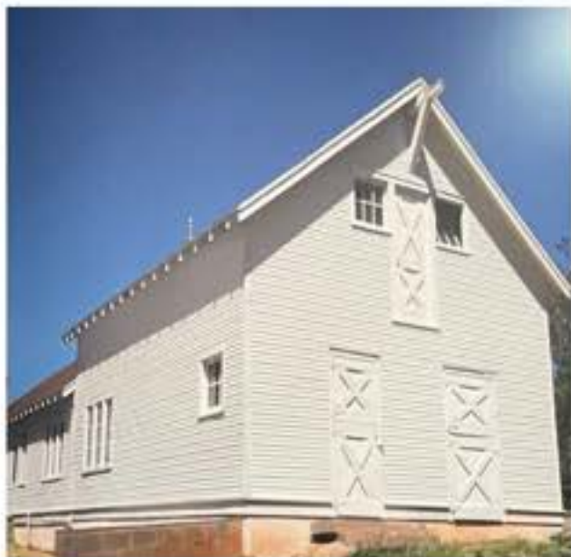
Ranger Station Barn
