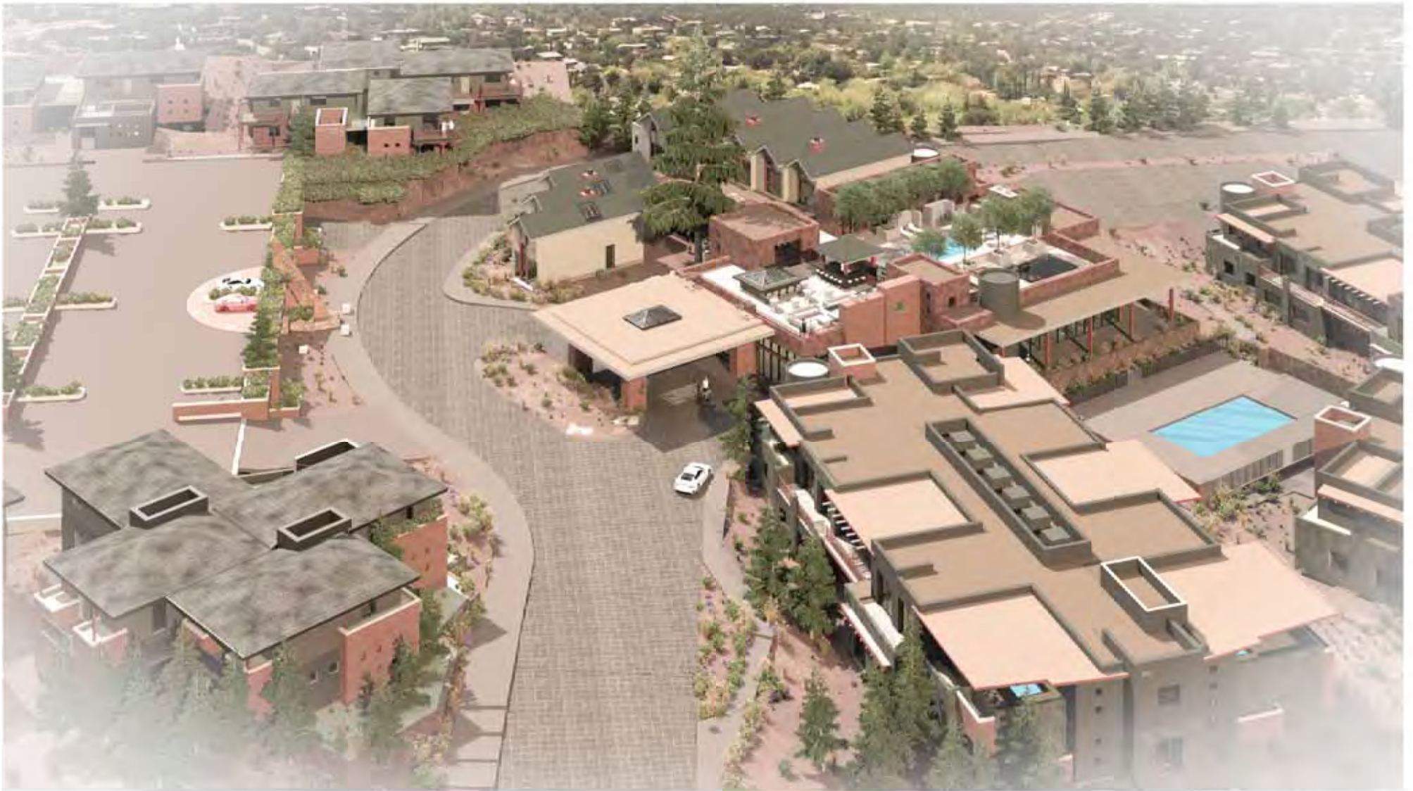
View from 89a looking south the Village at Saddlerock Crossing Soldiers Pass Road & Highway 89A Sedona Arizona Stephen Thompson Architect. Sedona/Del Mar Studio@StephenThompsonArchitect.com C: 928.301.5922 4/18/2021
