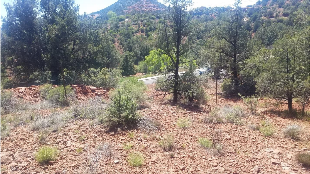
Figure 3: General site conditions showing the presence of over-sized aggregate (greater than 3.0 inches)
