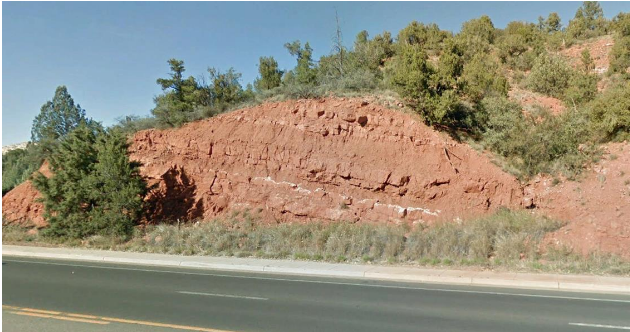
Figure 7: Cut slope at the base of the site – North side of Hwy 89A (Psm – Permian Supai Group)
