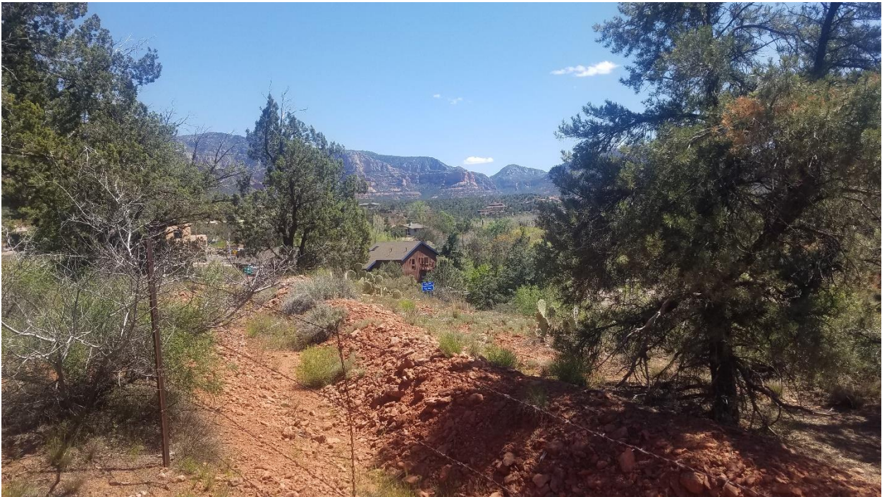
Figure 4: General site conditions showing the presence of over-sized aggregate (greater than 3.0 inches)
